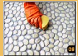
09 Repeat sponging off the grout until the desired look is reached. Once the grout has completely cured, seal the tiles with a good quality penetrating sealer. Color and shine enhancers can also be applied to vary the finish of the stones.
