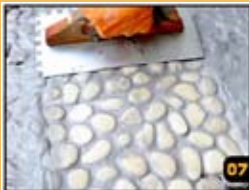
07 Remove the grout on the surface of tiles.
