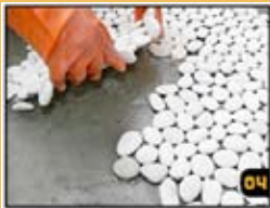
04 Set each tile close to the others on the thinset mortar. Lightly tap down the tiles without pushing the stones into the thin set cement. Wait the interval recommended by the mortar manufacturer before sealing and/or grouting to avoid dislodging the stones.
