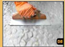
06 Apply a sanded grout on tile sections until the entire surface is covered.
