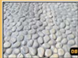
08 Prepare sponging off the grout. While wait the grout goes down to the edges of the tile.
