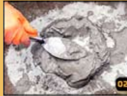
02 Use a high quality thinset mortar.
