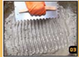
03 Apply the thinset mortar with a 1/4" notched trowel. It is strongly recommended that waterproof membrane systems are used in all wet areas.
